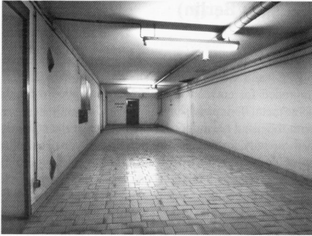
Shelter. under the station.
